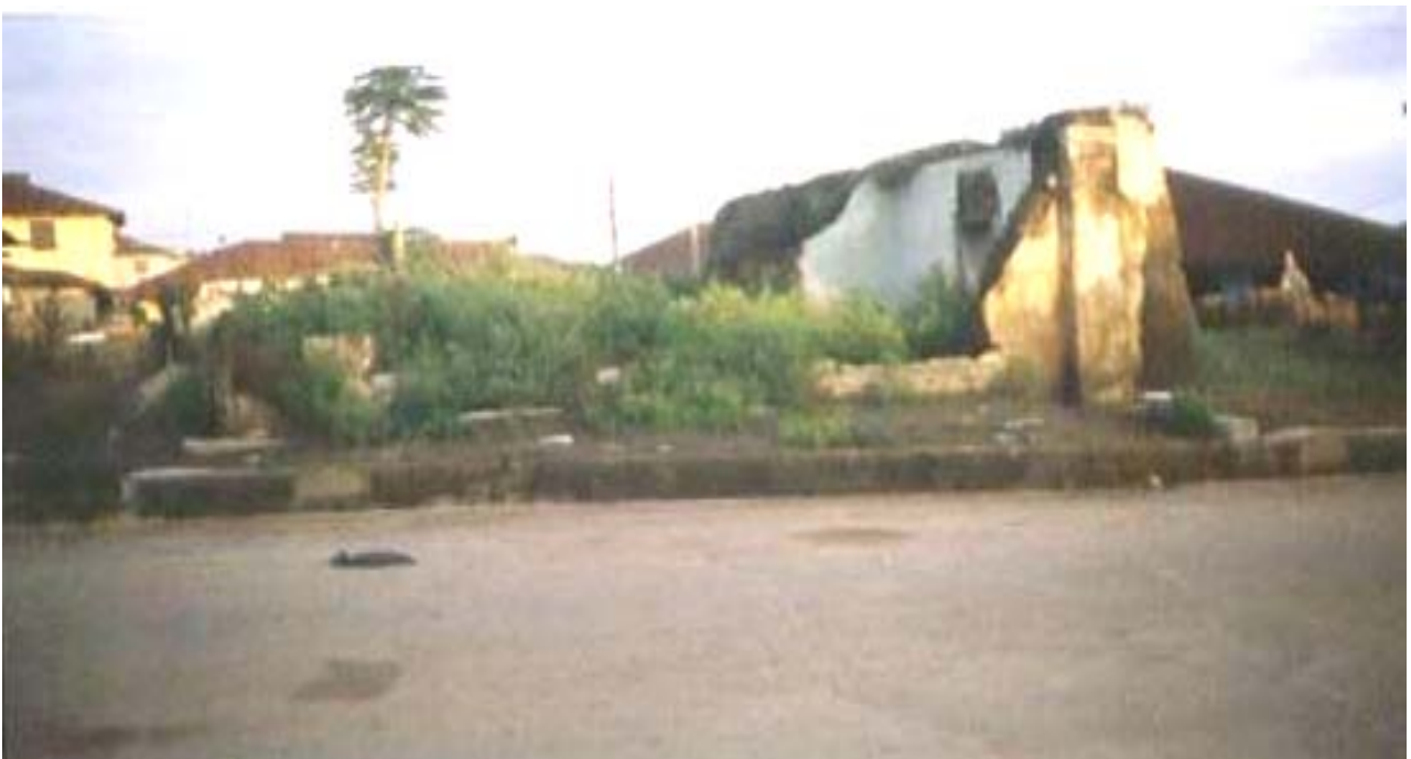
Plate 1b: Collapsed building left uncared for in the study area Source: Field Survey, 2010
