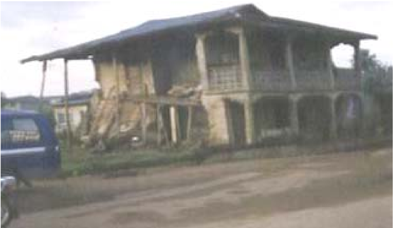
Plate 1a: Collapsed building along Odokoyi still inhabited by people due to high level of poverty. Source: Field Survey, 2010
